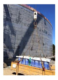
The application of crystalline waterproofing was completed in September 2014. Construction of the reservoir is scheduled to be completed by February 2015.
